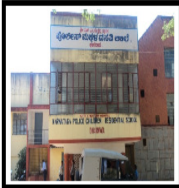
Picture 2: N A Muttanna Memorial Police School, Dharwad, Old Building
